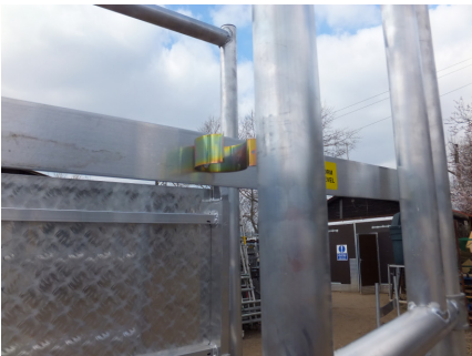
5. SWING GATE AND LOCK GUARDRAIL HOOK ON TO THE VERTICAL OF THE FRAME BEFORE COMMENCING WORK.
