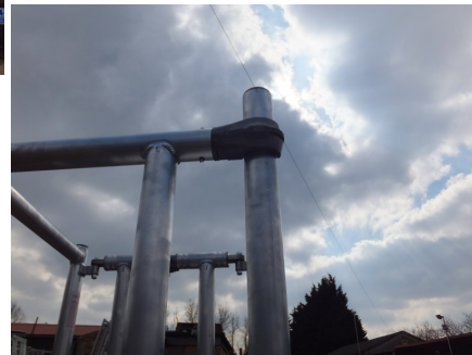
5. SWING GATE AND LOCK GUARDRAIL HOOK ON TO THE VERTICAL OF THE FRAME BEFORE COMMENCING WORK.
